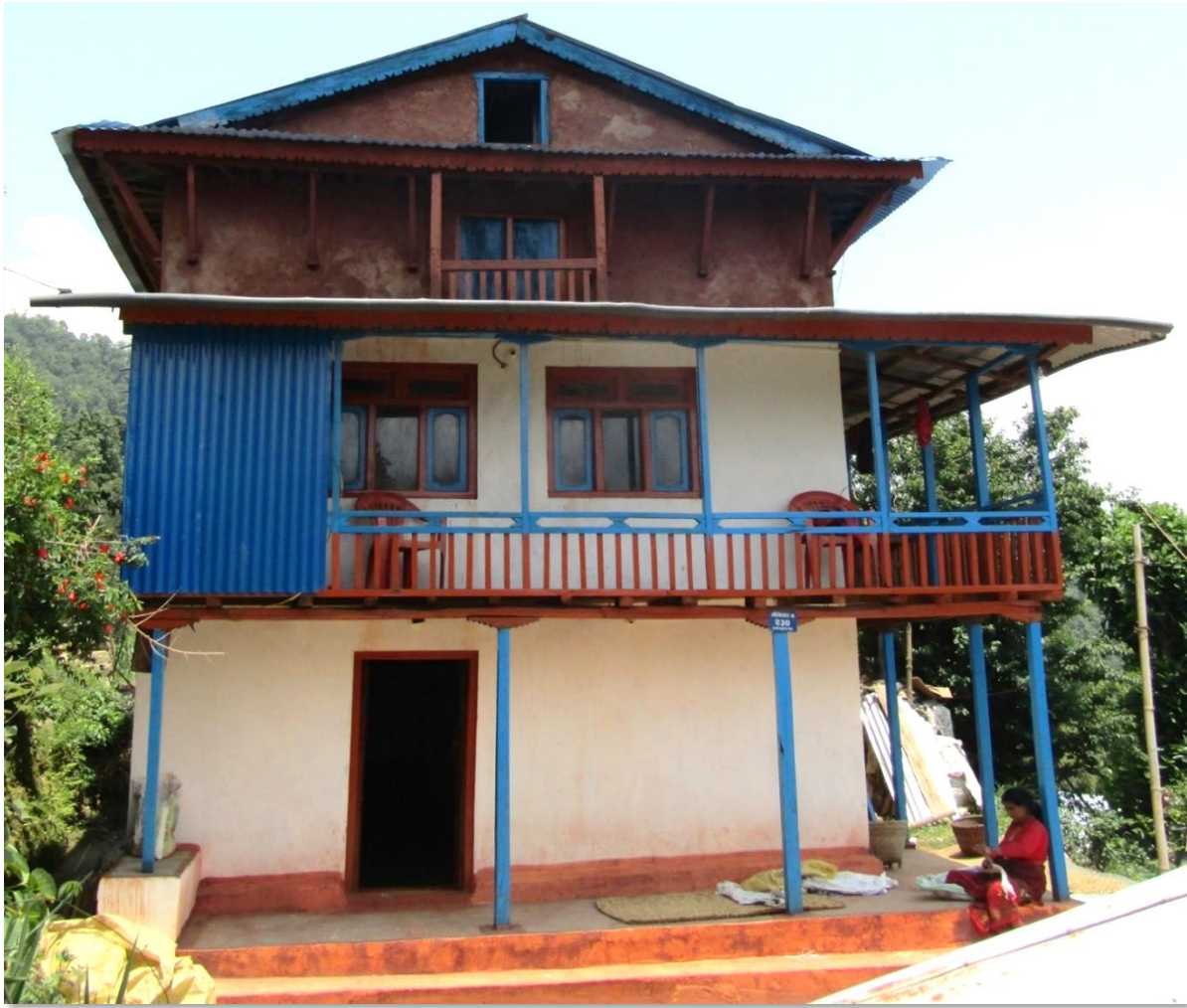
Retrofitted house, Dolakha
