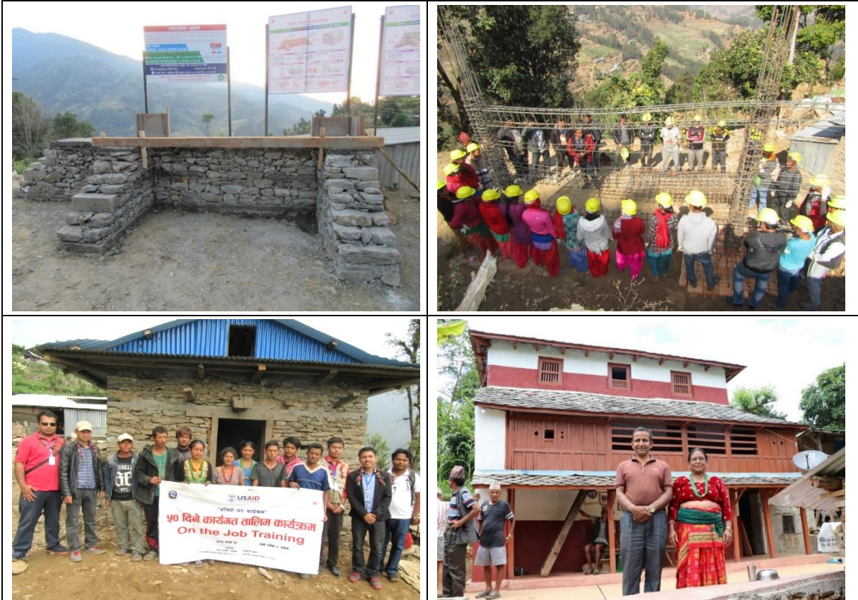
Demonstration Construction: Small Scale, Full Scale and Retrofit
