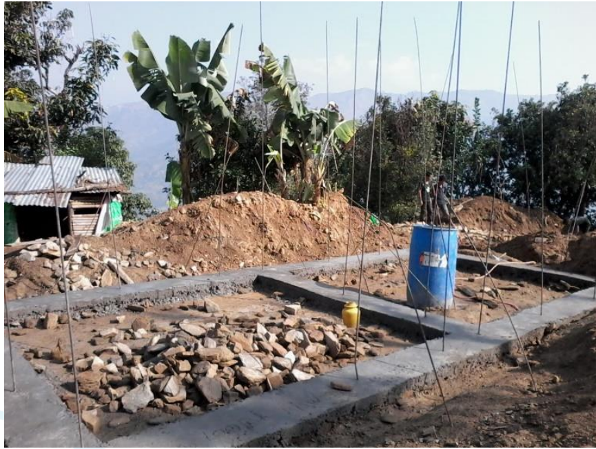
House of Ms. Sita Devi under construction
