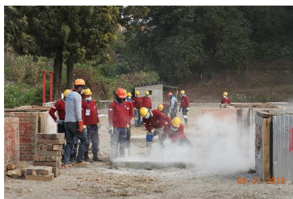
CSSR: Cutting concrete using Rotary Rescue Saw
