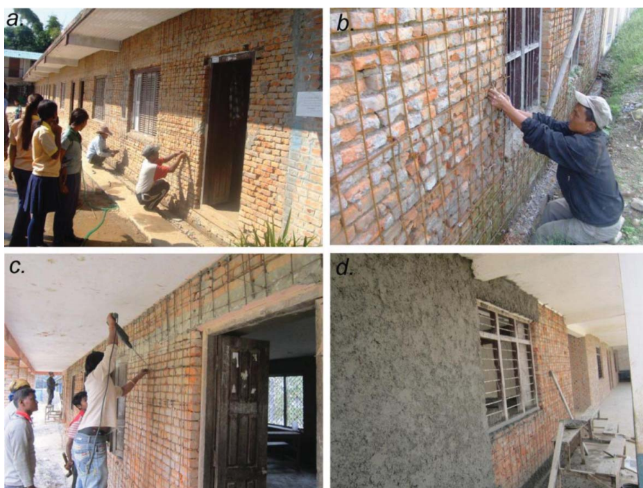
Figure 11. Retrofitting of school buildings in progress: (a) Gorakhnath Secondary School, Kirtipur, Kathmandu (jacketing on the wall with steel reinforcement), (b) Janaudah Lower Secondary School, Lalitpur district, Kathmandu valley (close view of steel reinforcement placing), (c) Chundevi Higher Secondary School, Kathmandu (steel reinforcement anchoring to the wall), (d) Saraswati Secondary School in Thecho, Lalitpur district, Kathmandu valley (micro concreting after steel reinforcement).
