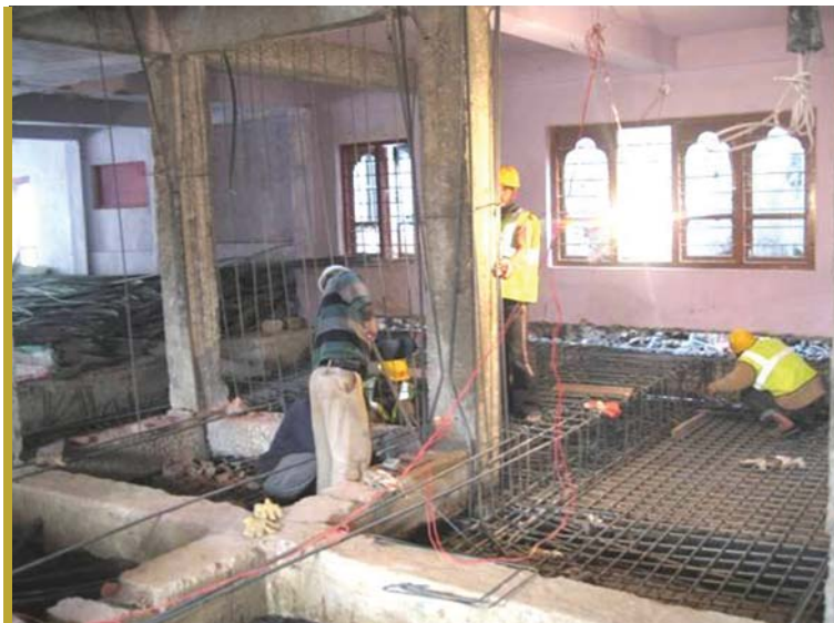
Work in Progress, placing reinforcement bars on raft, beam, column and shear walls
