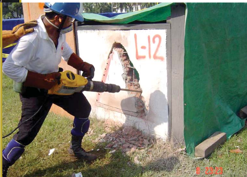
Breaching concrete during CSSR course
