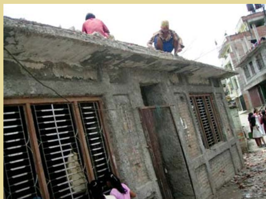
Retrofitting work undergoing at Buddha Jyoti Bal Udhyan LSS, Balaju under SESP/DRRSP of Action Aid Nepal
