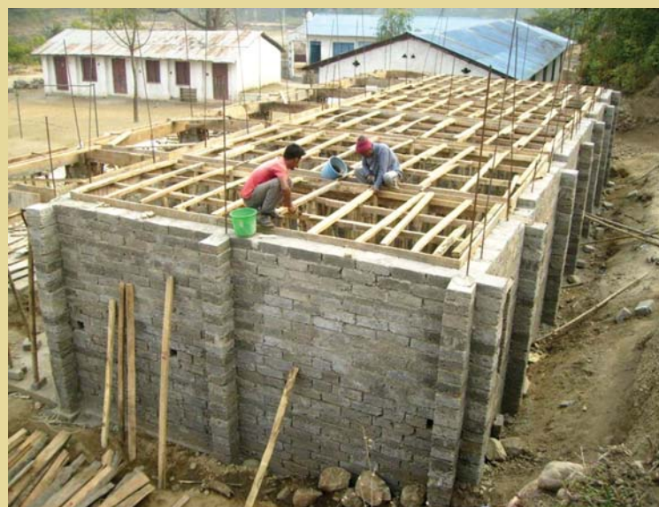
Construction work of school building of Marsyangdi Lower Secondary School, Lamjung is ongoing under GFDRR/The world Bank
