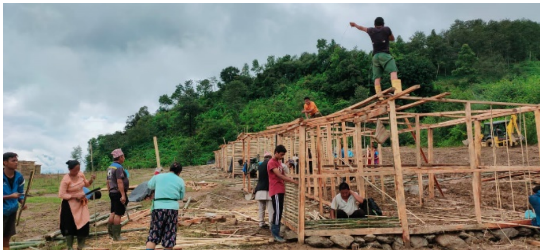
Villagers working for wood and Bamboo centibera skeleton construction.
