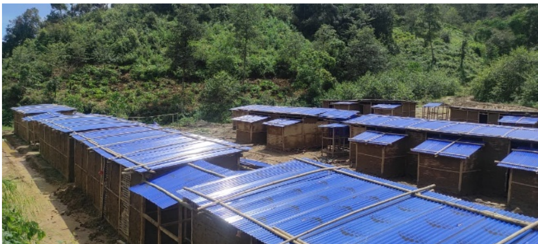
Overview of the shelter after roofing and mud plastering
