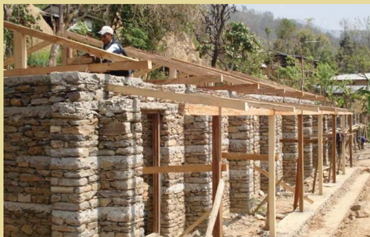
Construction work of School building of Bagishwori Secondary School, Lamjung is under going under GFDRR/The world Bank
