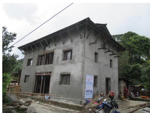
House of Purusartha Shrestha after retrofitting the house
