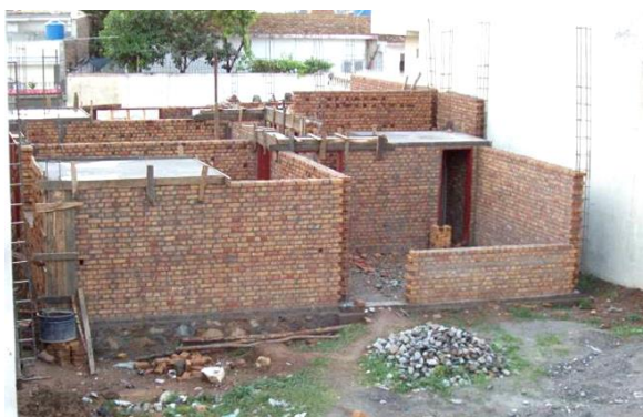
Construction sequence of confined masonry
