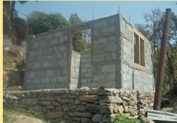
Reconstructed house of Ms. Yogi at lintel level
