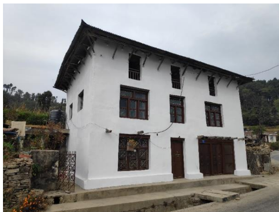
House of Ananda Bahadur Shrestha after retrofitting the house
