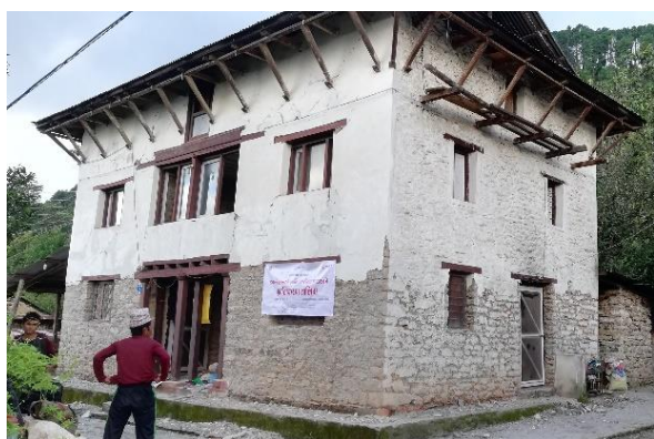
House of Purusartha Shrestha before retrofitting the house
