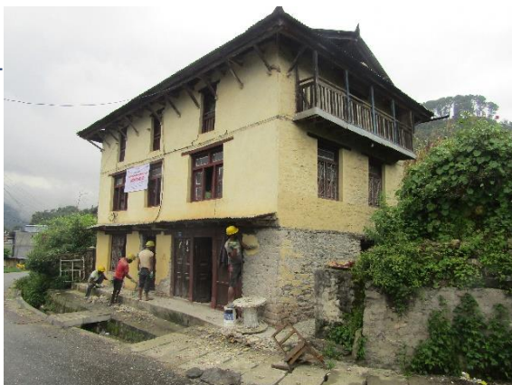
House of Ananda Bahadur Shrestha before retrofitting the house
