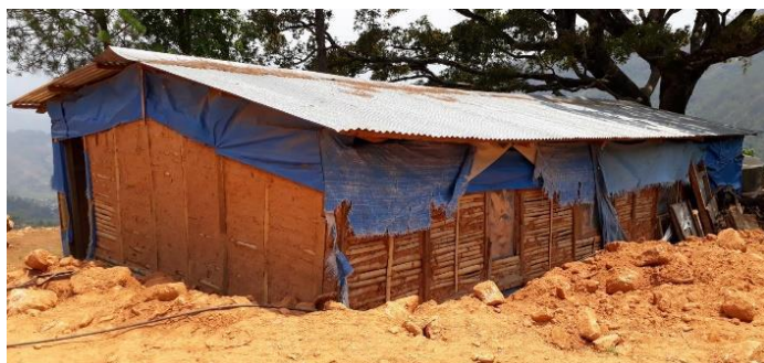
Chandra Nayan Basic School before construction
