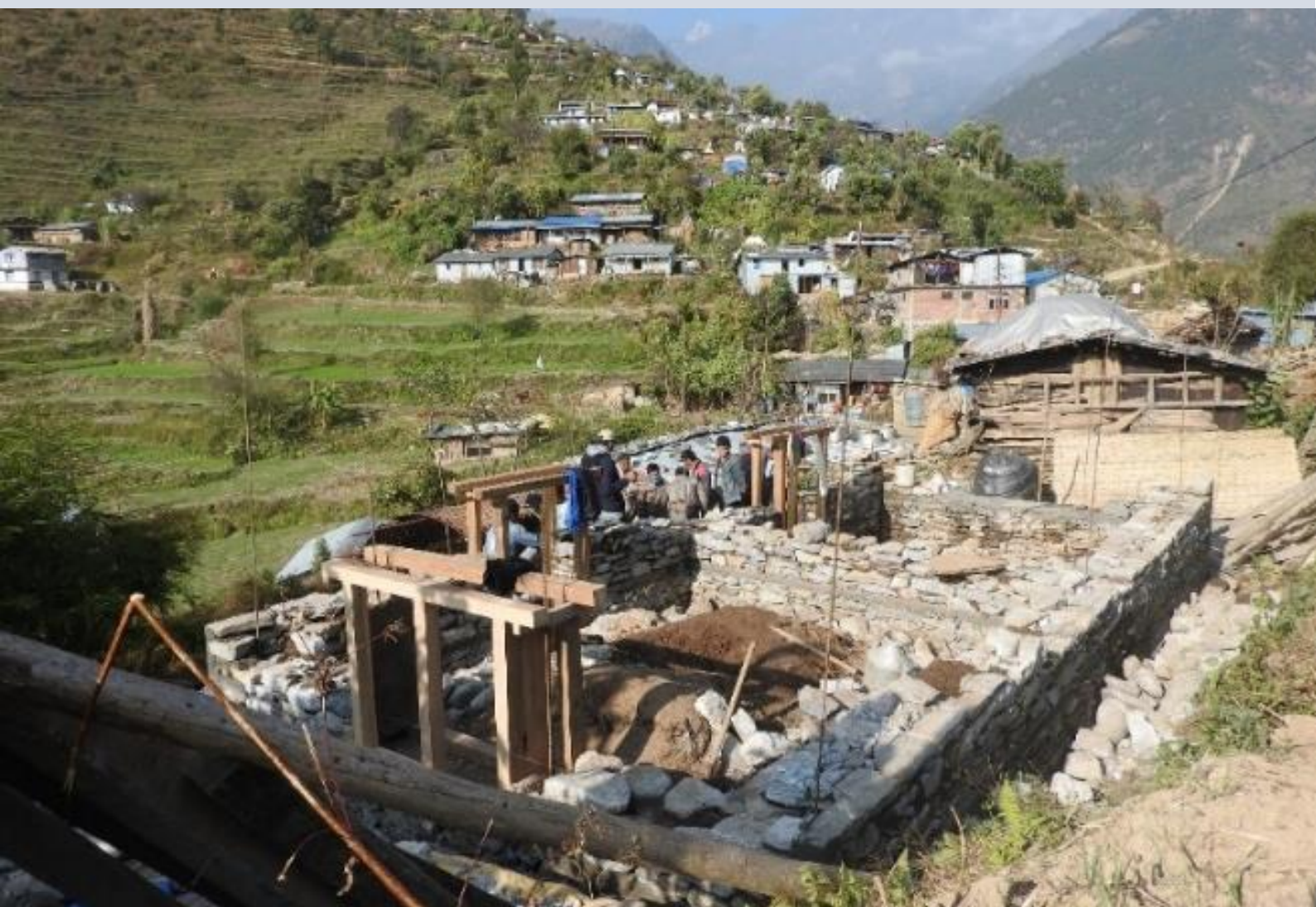
Aalampu being built better and safer
