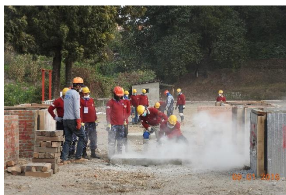
CSSR: Cutting concrete using Rotary Rescue Saw
