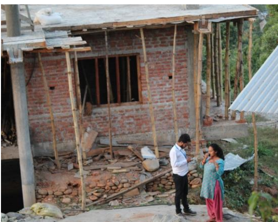
Conducting Building Compliance Survey
