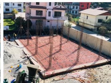
4. Placement of raft foundation reinforcement
