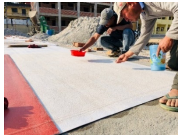
2. Filler sand laid on top of PVC
