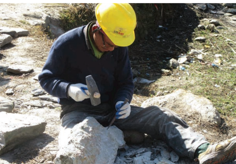
Mason dressing the stones to use in demonstration model likely to be built during practical exercise of Mason Training conducted at Tipling VDC of Dhading on 13th December 2016. Photo: BaliyoGhar
