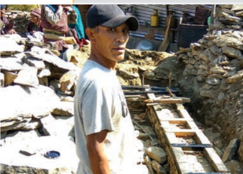
Mr. Sashiman Ghale preparing the plinth band
