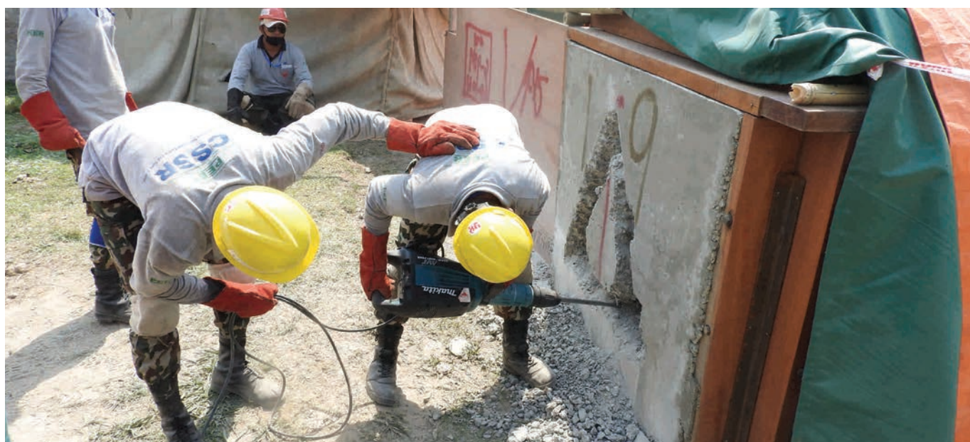
Participants of Collapsed Structure Search and Rescue (CSSR) training in practical session
