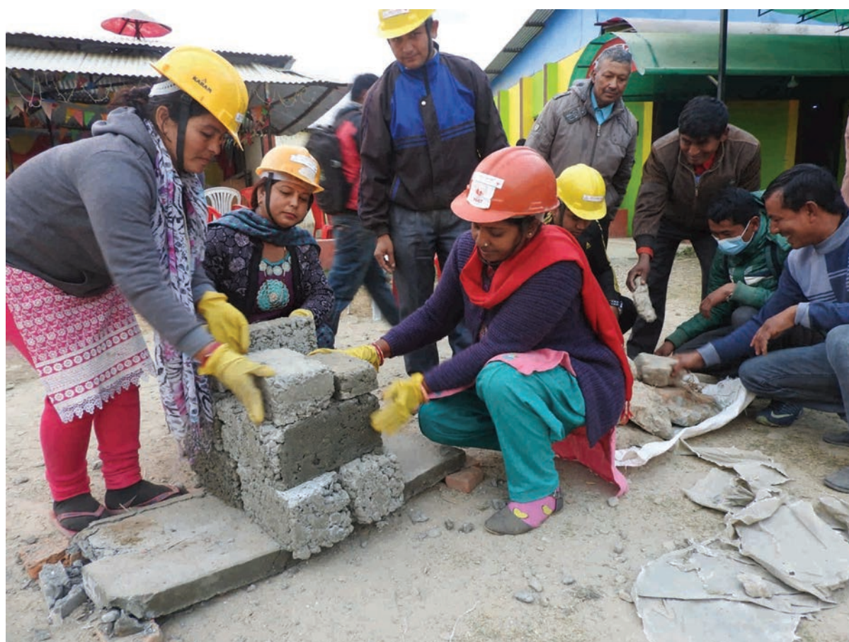
Female masons testing the slab prepared during the Mason Training at Kageshwori Municipality, Kathmandu in December 2016. BaliyoGhar is providing technical assistance in Kageshwori Manohara Municipality of Kathmandu. Photo: NSET/BaliyoGhar
