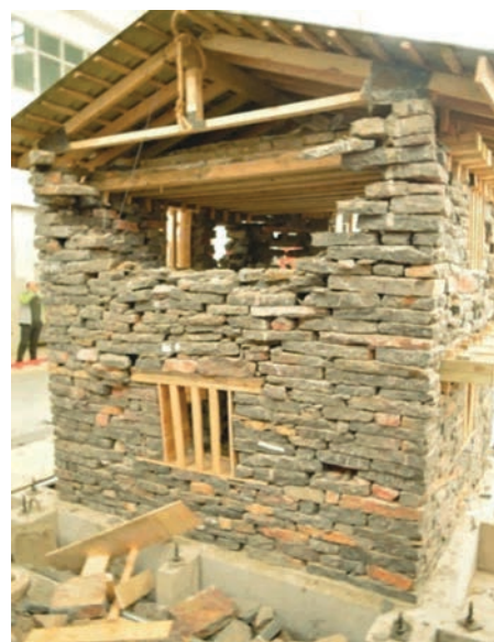
Unreinforced Masonry: Damage in Shake Table Test @ 0.4 g
