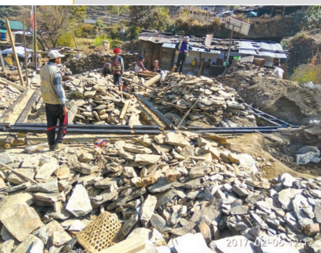
Treated Timber used as plinth band
