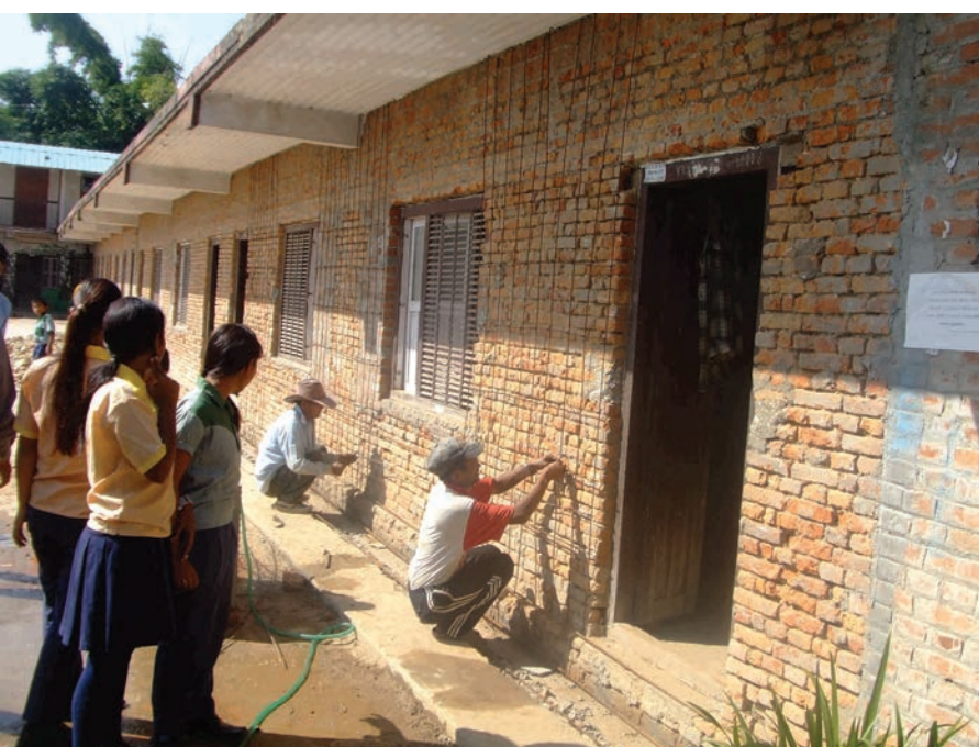
Retrofit of school building in progress, SESP, NSET
